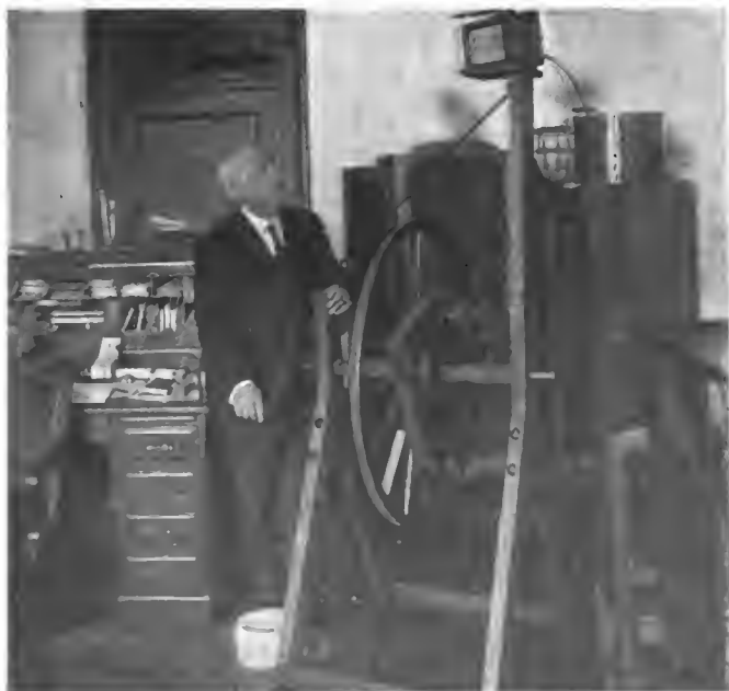
Col. Haskell and His Taximeter Testing Device at Work
